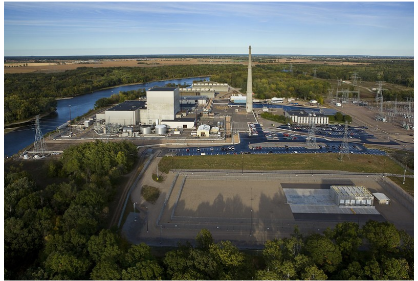
Photo courtesy of NRC Monticello nuclear plant
