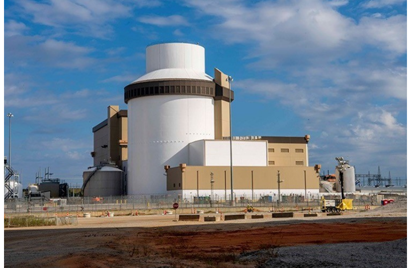
georgiapower.com Vogtle unit 3
