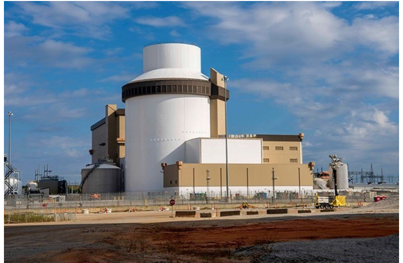
georgiapower.com Vogtle unit 3
