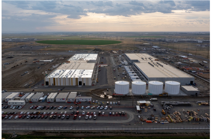
AP Images Amazon Web Services data center
