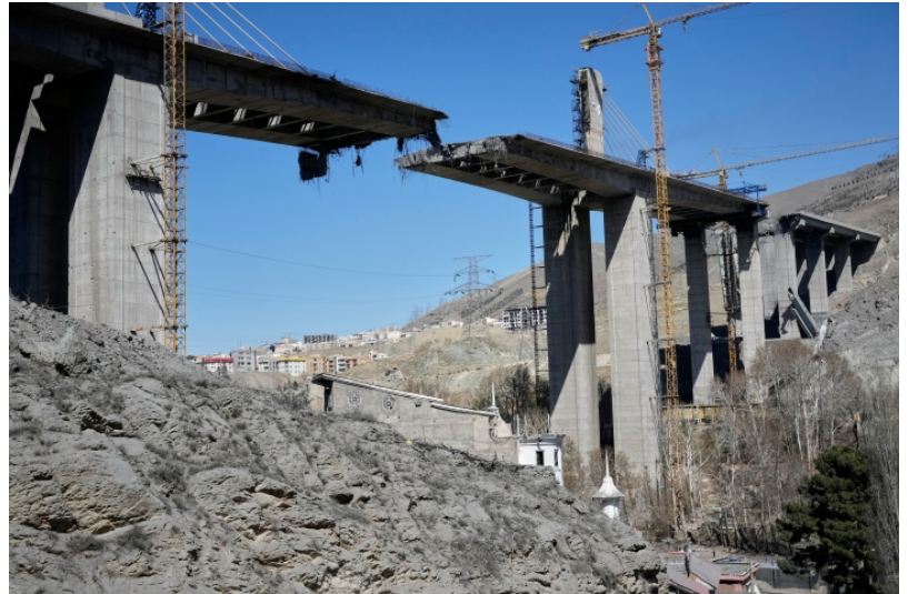
AP Images B1 bridge outside Tehran, Iran
