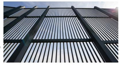
It will be at least 18 feet in height, but CBP's "nominal" goal is more like 30 feet above ground, and another six feet below ground (to discourage tunneling underneath it). It's also going to be thick, as one of the requirements is that it must take someone at least an hour — and ideally more than four hours — to bore a hole in it large enough to allow him to crawl through it. That, theoretically at least, would allow enough time for border agents to respond to the effort.
