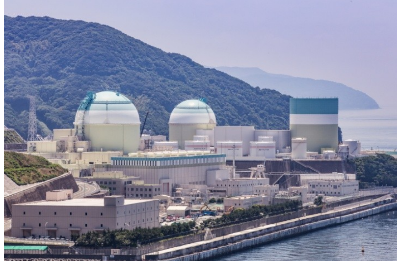
paprikaworks/iStock/Getty Images Plus Ikata nuclear power plant (Ehime Prefecture) in Japan
